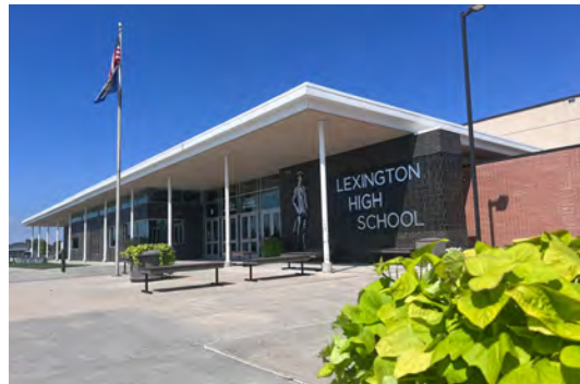
Figure 59: Lexington Senior High School Lexington Senior High School 13th Street and Adams Street
