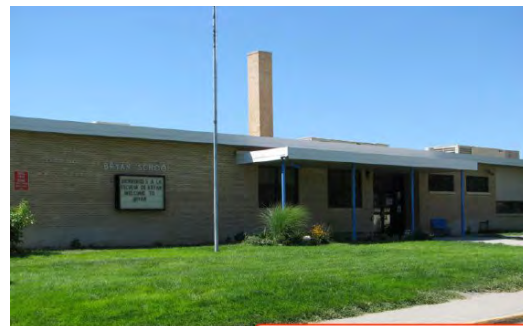
Figure 55: Bryan Elementary School Bryan Elementary 11th Street and Harrison Street
