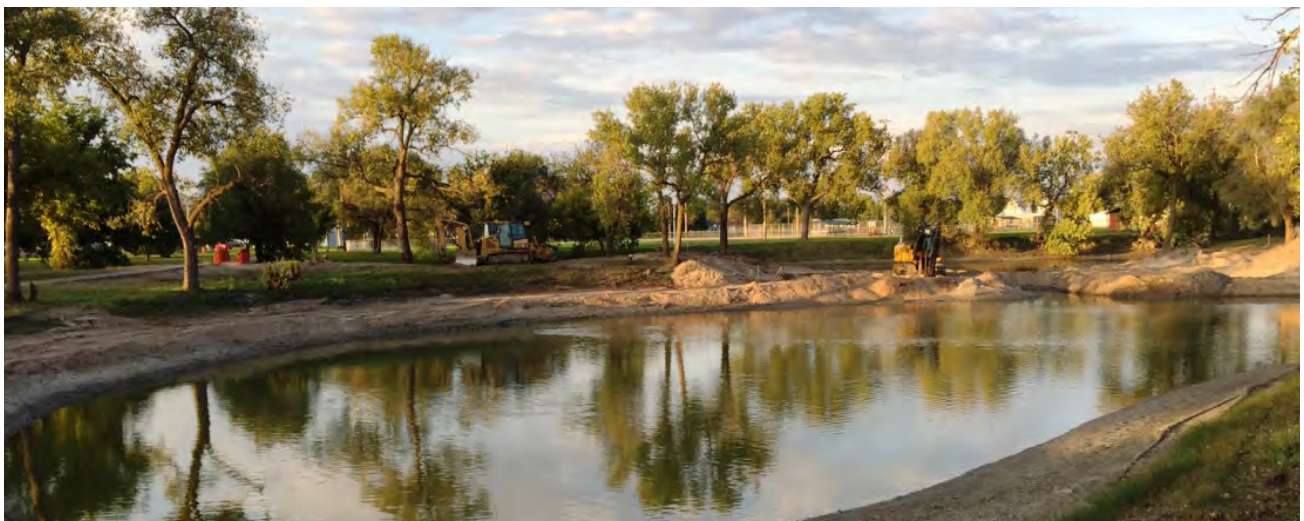
Plum Creek Park lake restoration project construction.
