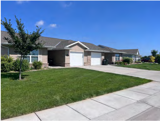
Newly constructed Age In Place housing development.
