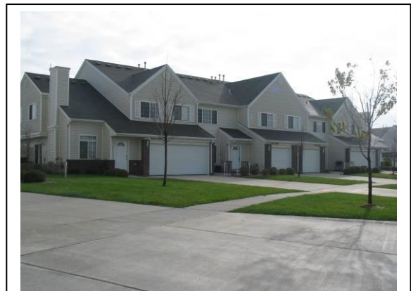
Example of Single-Family Attached
