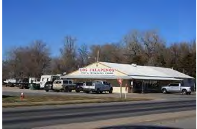
Older Restaurant Building.
