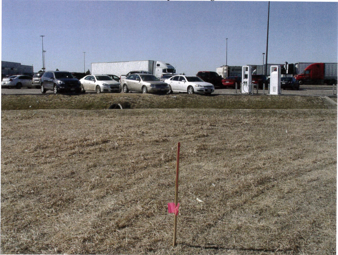
Location of Monopole looking West
