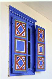
Both interior and exterior, can help reduce summertime heat gain in your home. Remember that interior shutters need a clear space to the side of the window when they are opened. They also require hardware that is fastened to the window jams or trim. Properly designed exterior shutters may provide the best possible window insulation system. They also offer advantages of weather protection, added security, and no use of interior space.
