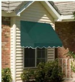
With their recent rise in popularity, the U.S. Department of Energy calculates that window awnings can reduce solar heat gain in the summer by up to 65 percent on south-facing windows and 77 percent on west-facing windows. Today, awnings are made from synthetic fabrics that are water-repellent and treated to resist mildew and fading. You should choose one that is opaque and tightly woven. And be aware that light-colored awning will reflect more sunlight than a darker awning.
