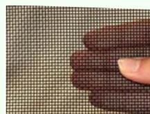
Mesh window screens can diffuse solar radiation, reducing heat gain in
