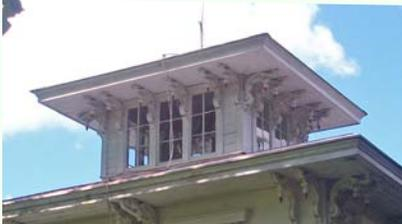
Properly sized and installed roof overhangs can most effectively shade south-facing windows from summer heat. If oriented properly, overhangs will allow sunlight through the windows during winter, providing more warmth to a house.
