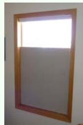
An insulating window panel or pop-in shutter typically consists of a core of rigid foam board insulation. You can push or clip it into the interior of a window.
