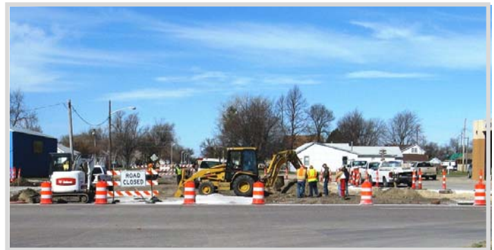
Walnut Street from Hwy 283 to Van Buren: complete removal & replacement
