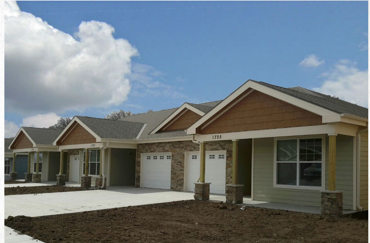
Newton, KS (taken while under construction)
