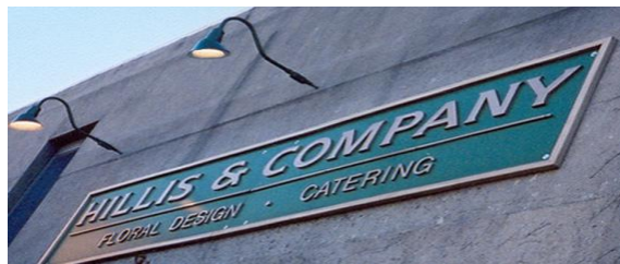
Example of a flush mounted sign panel located on the side of a building. This sign has raised letters and a simple color scheme. It is also lit with gooseneck lamps
