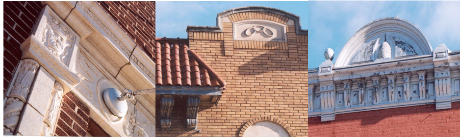
Terra cotta building detail on the Barmore Pharmacy Building; Stone detail on the IOOF Building; Beehive Building cornice detail.
