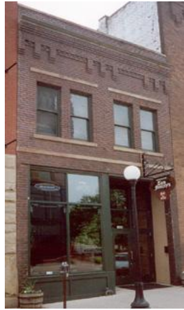
Appropriate storefront replacement. The style, size, proportions and materials are consistent with the original storefront.
