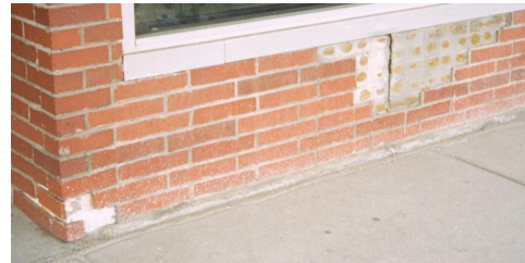
f. applied false brick veneer (a.k.a. z-brick)
