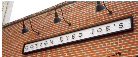
Example of good exterior lighting. The simple style of the lighting fixtures matches the simplicity of this simple commercial building.
