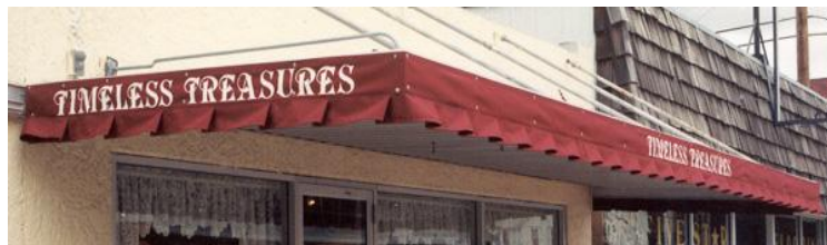
Example of a canopy skirt with signage. The lettering can be sewn directly onto the canvas or it can be screen-printed.
