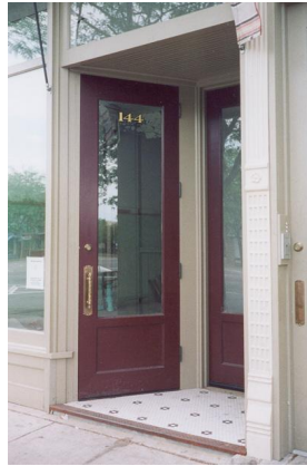
Example of an appropriate historic commercial door.
