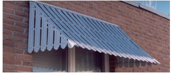
Metal stock awnings are not recommended. Example of a metal stock awning. These awnings are most commonly found on homes but have been applied to commercial buildings.
