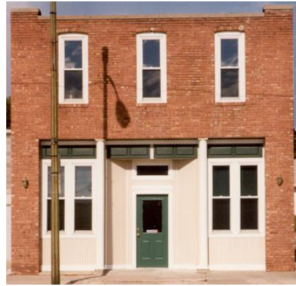
Inappropriate storefront replacement. The style, size, proportions, and materials are NOT consistent with the original storefront. The color selection is also inappropriate.
