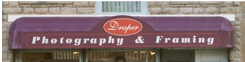
Example of a backlit plastic awning. This type of awning is unacceptable in the district.
