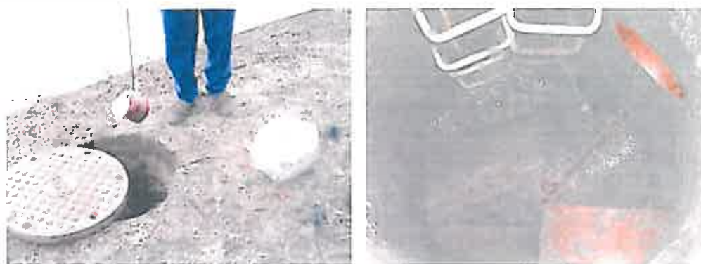
Figure 64: Dye in a mesh bag is placed into an upstream manhole (left); Dye observed at a downstream manhole traces the path of the storm drain (right)
