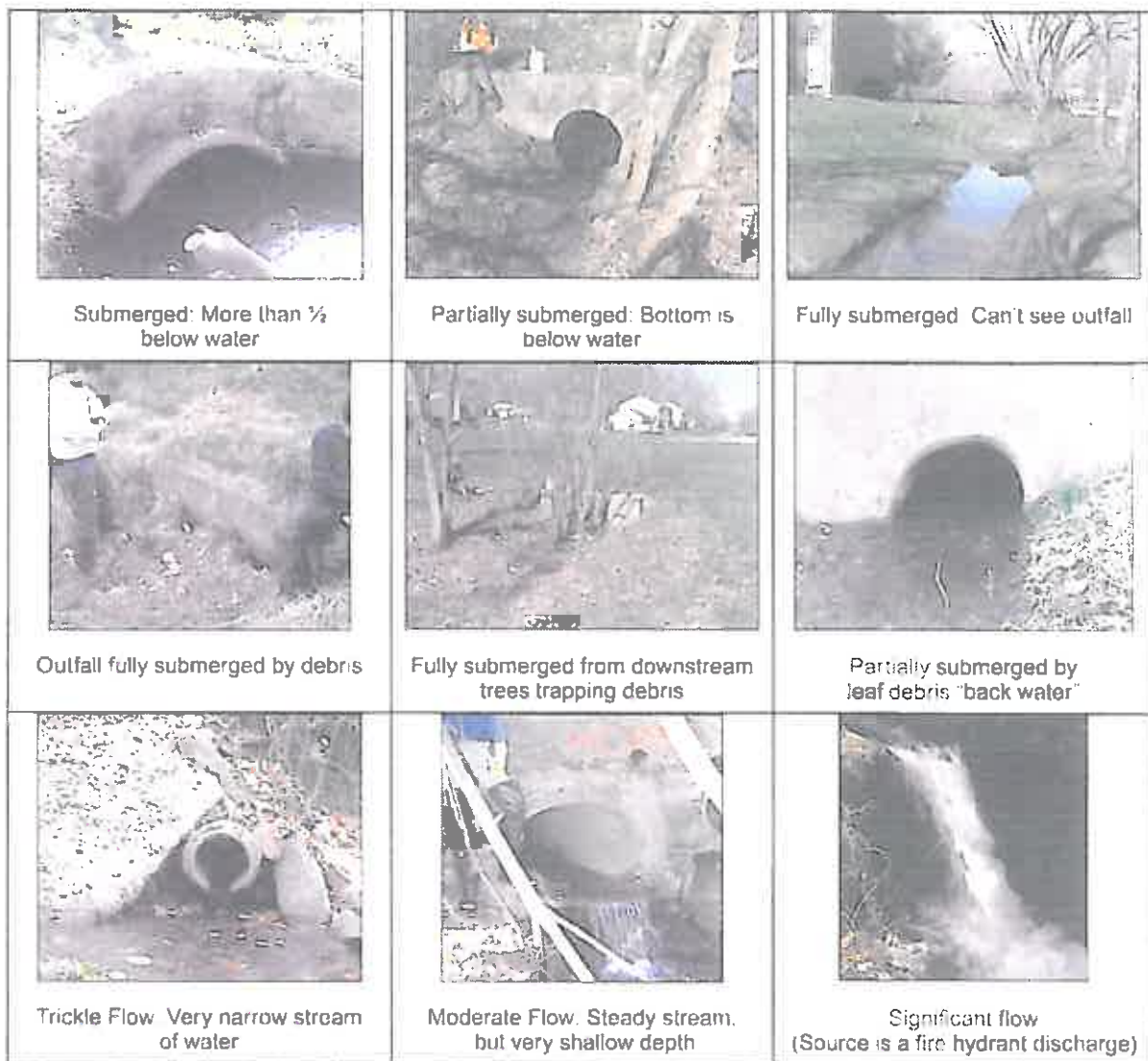
Figure 28: Characterizing Submersion and Flow
