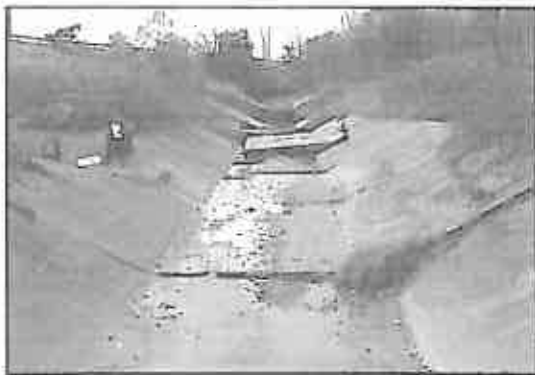
Figure 19: Walk all streams and constructed open channels
