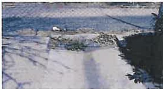
Debris and litter clog the drainage inlet and mix with storm water runoff.
