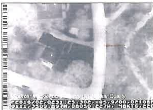
Figure 74: Aerial Thermography Showing Sewage Leak
