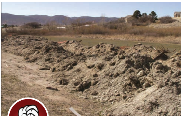
Fig. 4-6. Stockpiles left exposed need surface treatment.
