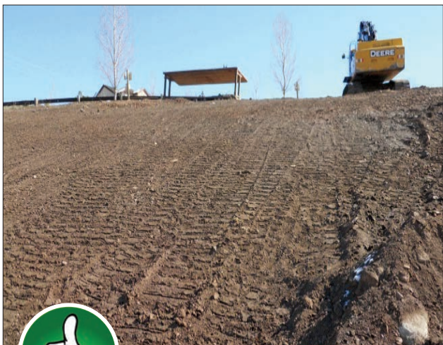
Fig. 4-5. Excellent example of proper tracking; tracks are perpendicular to the slope.
