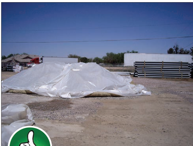
Fig. 1-9. Covering a pile and maintaining a low profile shape are good ways to reduce wind erosion potential.
