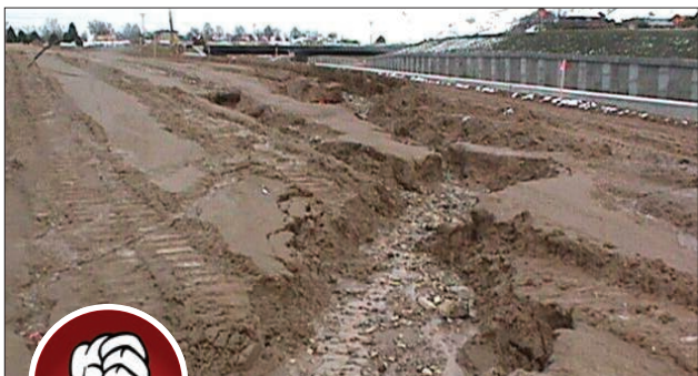
Fig. 5-18. Severe gully erosion such as this is a clear sign of the need for a temporary drainage system. Source: Utah DOT
