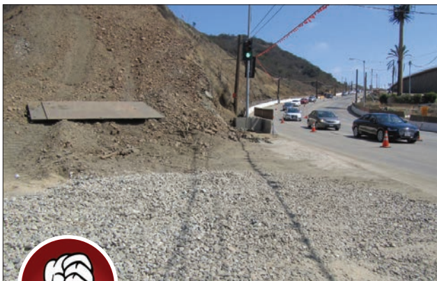
Fig. 3-13. The size and placement of rock is ineffective at controlling sediment at the project entrance. Larger rock combined with a filter fabric would help. Source: RBF Consulting
