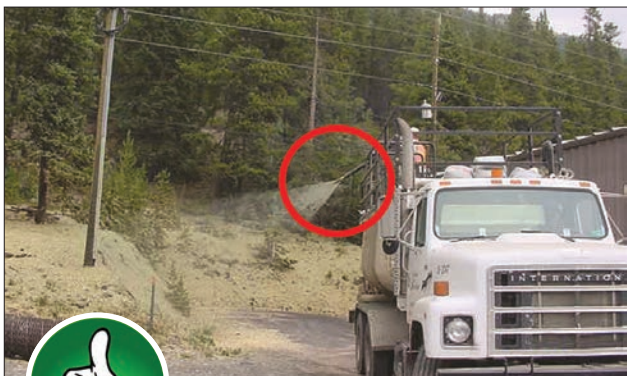
Fig. 4-7. This is a good example of tackifier application using a fan nozzle.
