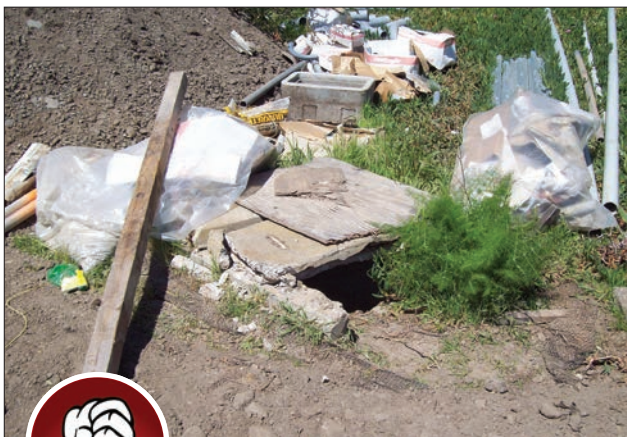
Fig. 2-1. Trash and debris are among those most common pollutants at construction sites. Proximity to open storm drains is especially problematic.
