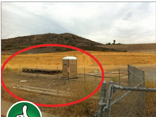
Fig. 2-2. This portable toilet shows no evidence of trash, debris, or drainage of liquid waste. Note the use of perimeter controls along the downward sides. Source: RBF Consulting
