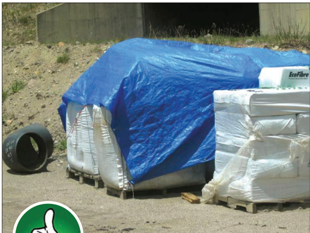
Fig. 2-4. Materials are being properly stored on pallets, and unused materials are covered with a tarp. Source: Colorado DOT
