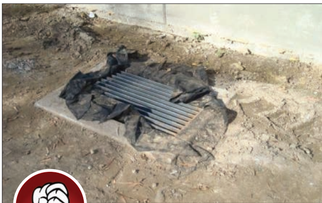
Fig. 5-13. Instead of filter fabric held in place by the grate, silt fence, sand bags or other sediment controls should be used to keep silt away from grate. Source: RBF Consulting
