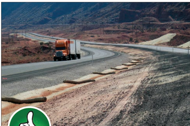
Fig. 5-23. This picture shows a good example of fiber roll check dams promoting settlement of fine sediment. Source: Utah DOT
