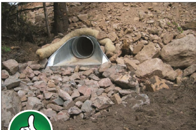
Fig. 5-28. The fiber roll above the culvert helps prevent debris and dirt from falling into the outlet. Source: Colorado DOT
