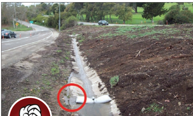
Fig. 5-22. Excessive spacing between check dams in this ditch and poor design and construction is causing flow to outflank the sides.
