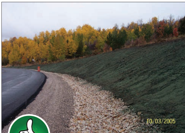
Fig. 4-11. The mulch application shown here has properly avoided the adjacent channel area.
