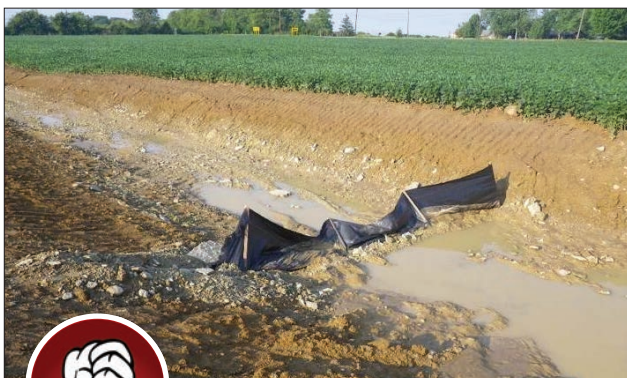
Fig. 5-21. Silt fence should not be used as a temporary check dam. Source: Ohio DOT
