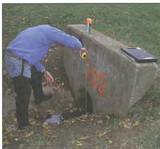
Figure 27: Measuring Outfall Diameter
