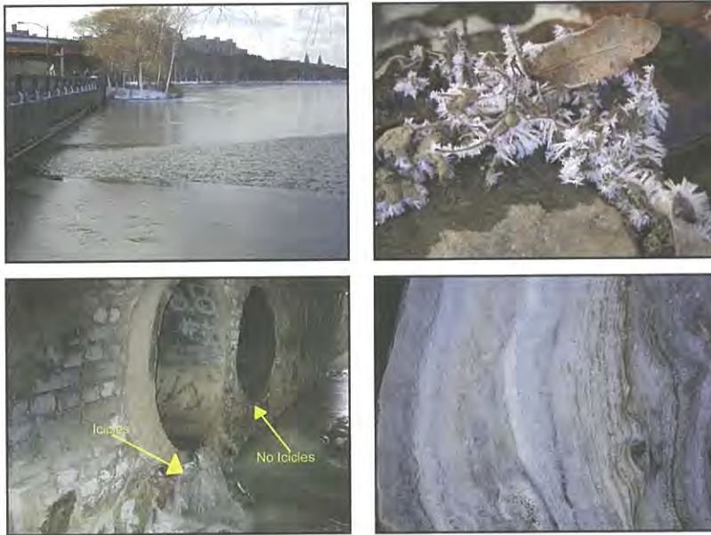
Figure 41: Cold climate indicators of illicit discharges
