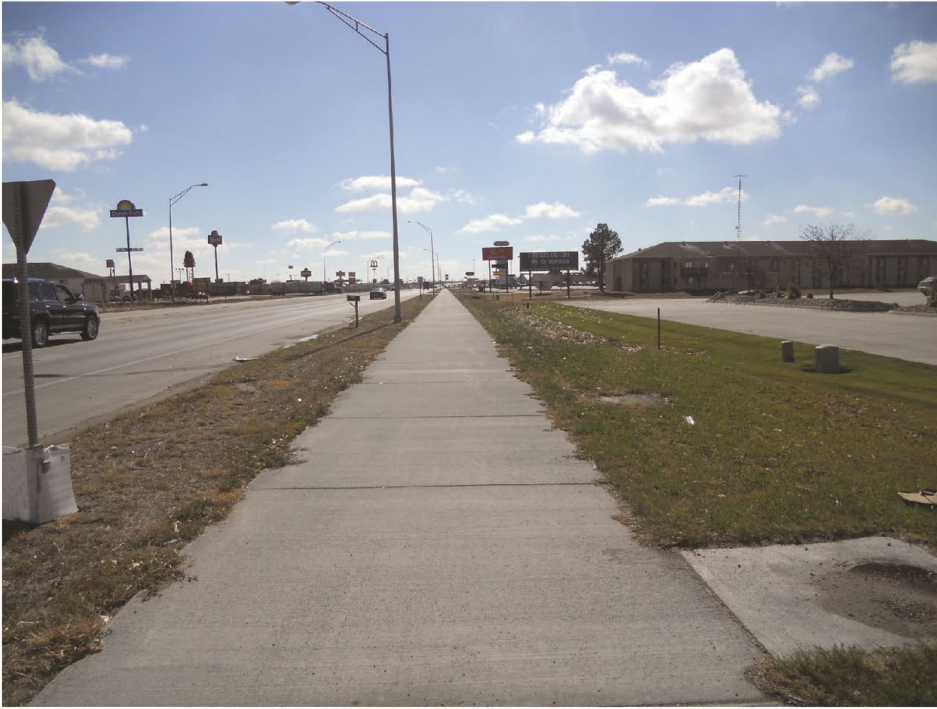
Existing Conditions along Plum Creek Parkway
