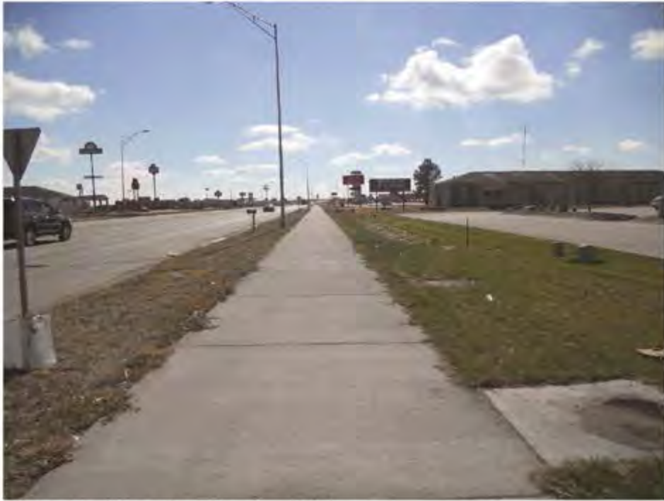
Existing Conditions along Plum Creek Parkway
