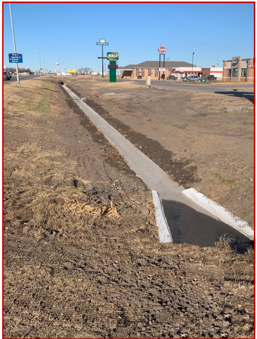
This new ditch flow liner is on the east side of south Plum Creek Parkway.
