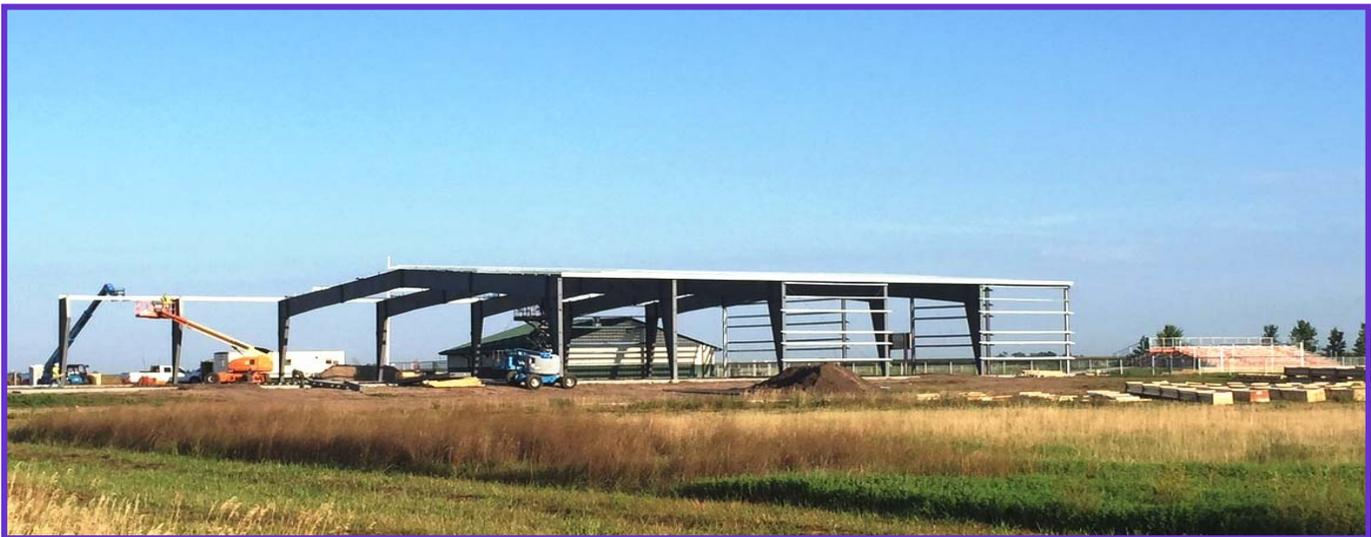
Lexington's new 27,000 square foot indoor activity center broke ground in mid-July with footing and foundation work. In early August, structural steel began rising from the ground. The long anticipated facility is planned to be operational by mid-October.
