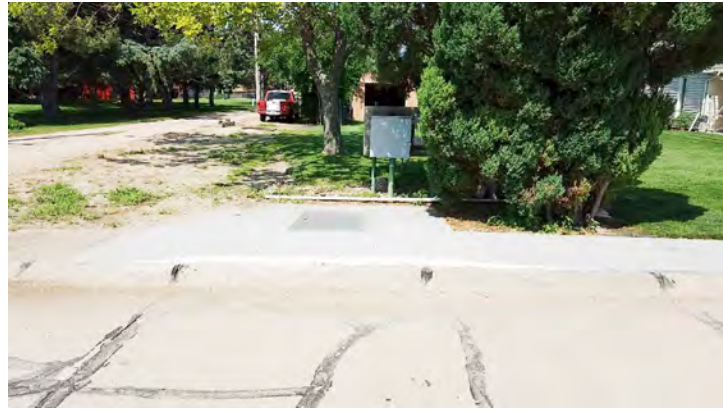
EXISTING LIFT STATION TO BE REMOVED
