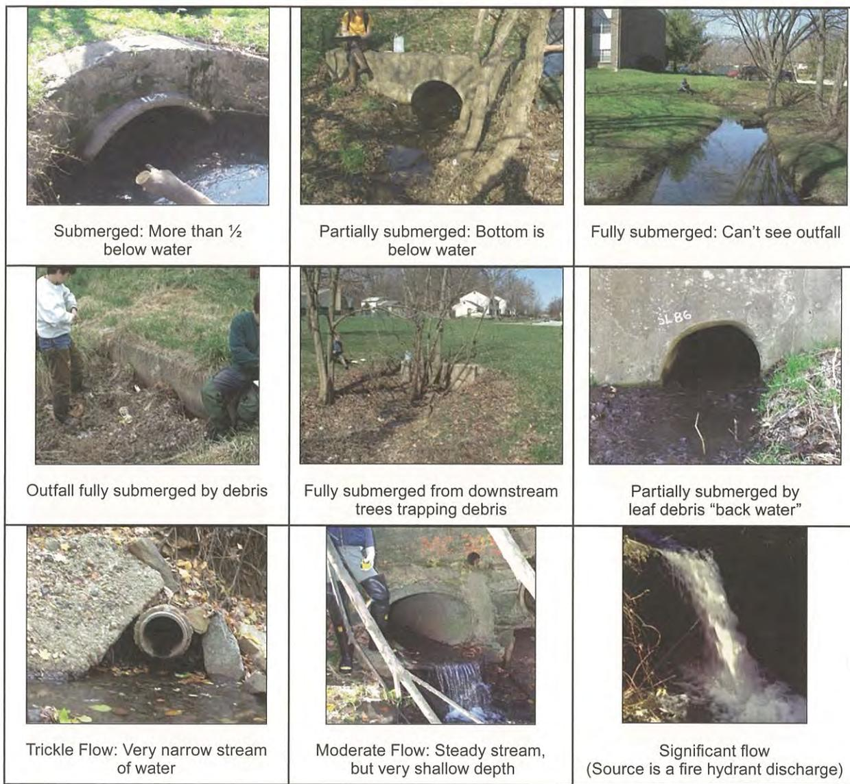
Figure 28: Characterizing Submersion and Flow
