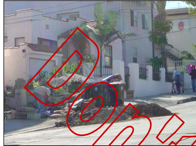
Don't stockpile dirt and other materials in the street.
